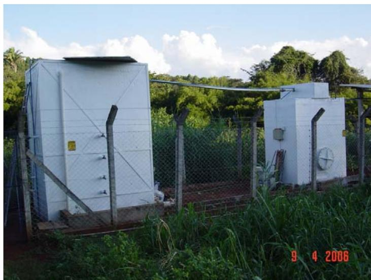
**FIGURA 12** Reator anaeróbio compartimentado (RAC) e reator UASB
